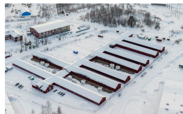
Data center in Boden, Sweden: PUE = 1.06 (2022)
