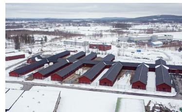
Data center in Boden, Sweden: PUE = 1.09 (2023)
